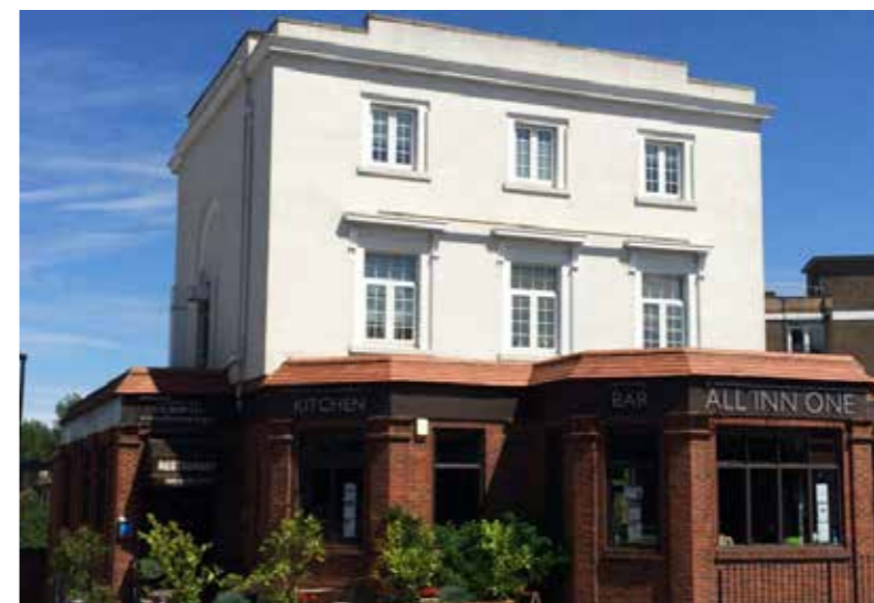
Fig. 7 – Photo of the West facade - 2017
