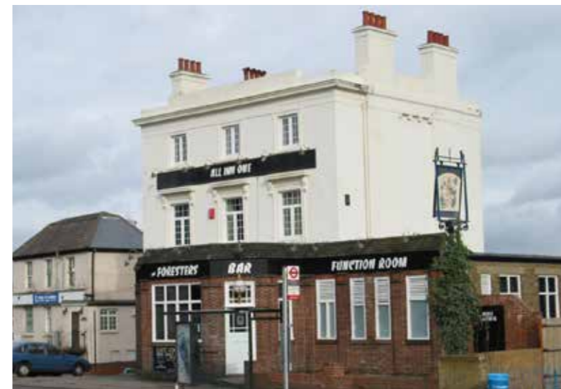
Fig. 6 – Photo of the West facade - 2003
