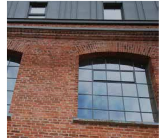
Fig. 20 – Crittal style windows
