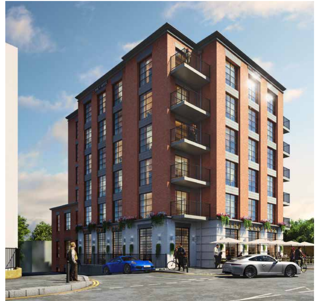
Fig. 9 – Design option with redbrick on the upper floors and white glazed brick to the ground floor
