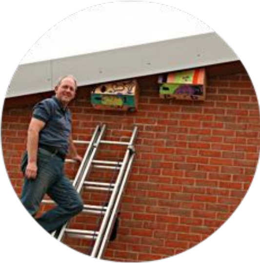
Installing boxes at a school. Copyright © Clarke Brunt
